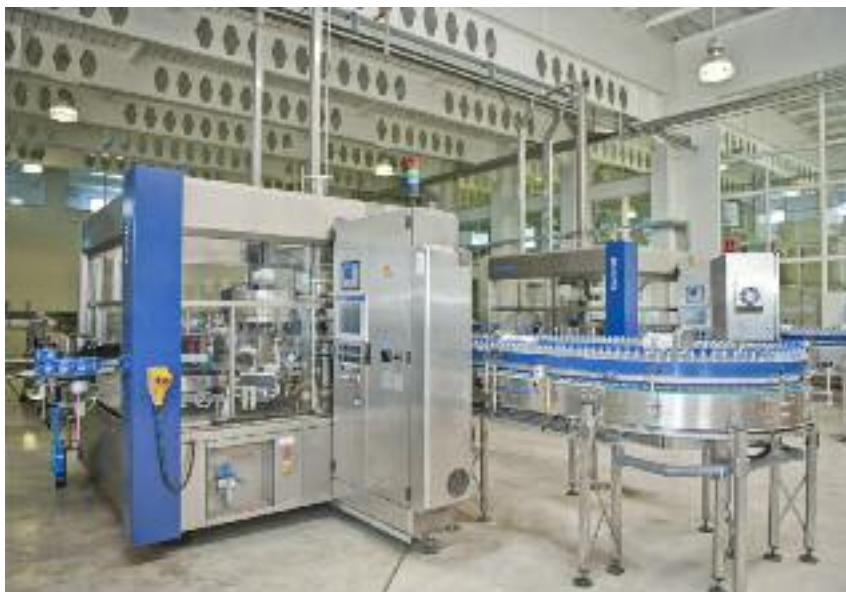
Outside the cleanroom, two Controll machines dress the 600ml and 1.500ml containers in wrap-around labels.
